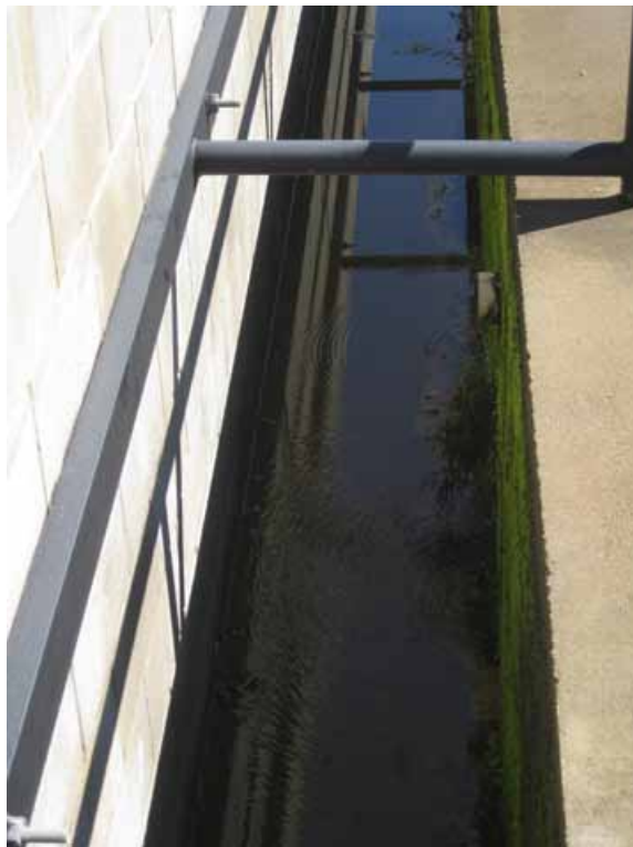
Figure 4. Algae growing in a facility's irrigation canal will introduce algae back into irrigation ponds.
